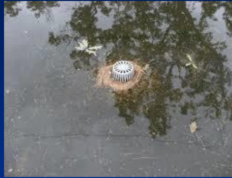
Ponding/drainage
