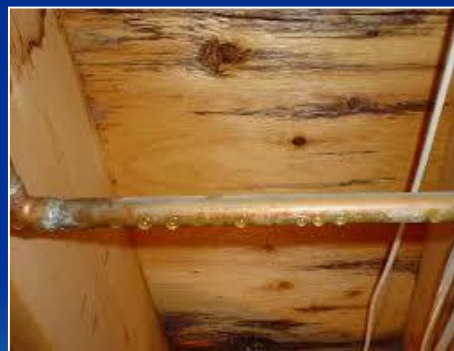
Piping Condensation
