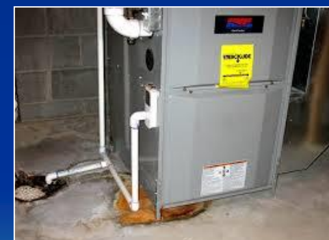
Condensate drainage
