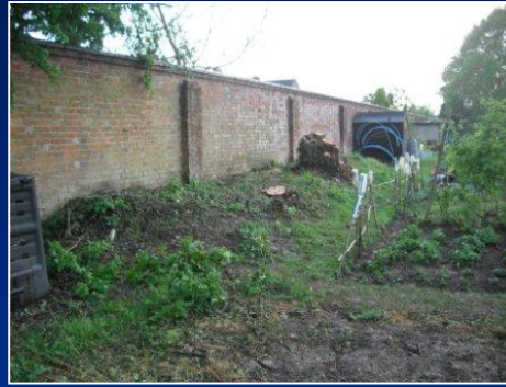
Soil abutting building
