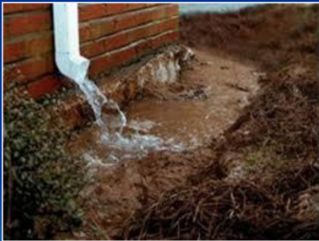
Downspout drainage
