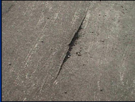
Lap/seam failure
