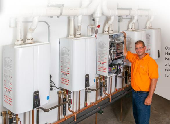
Contractors recommend Navien for its stainless steel heat exchanger. "It will last a lot longer than copper heat exchangers on other tankless units."
