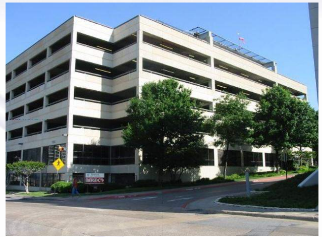
Parkland Healthcare System, Dallas, Texas Building Envelope Emergency Center Parking Garage
