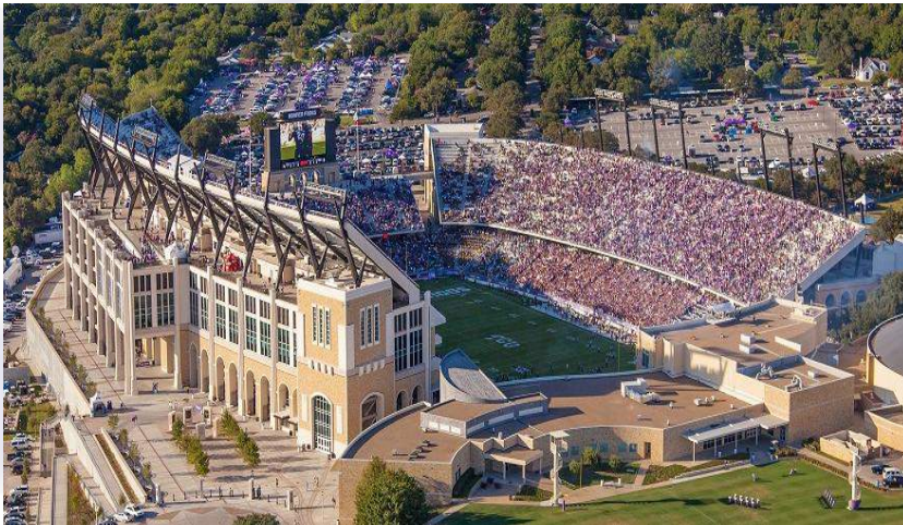
TCU Amon G. Carter Stadium Water Infiltration
