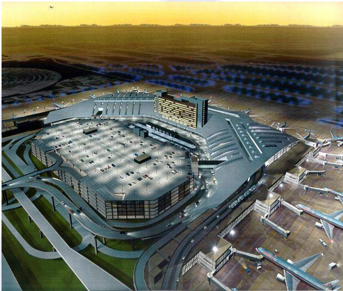
DFW International Airport, DFW, Texas Roof/Wall Program Management
