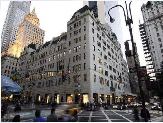
Bergdorf-Goodman, New York, NY Roof Replacement Design/Administration
