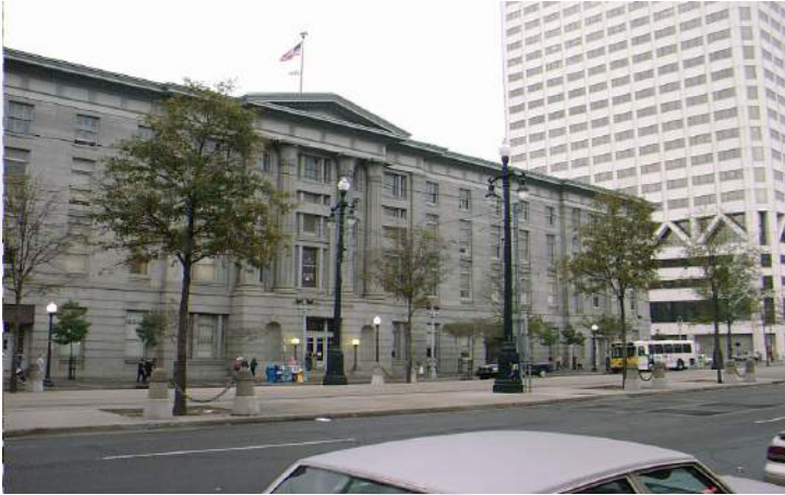
GSA Federal Buildings, New Orleans Hurricane Damage Assessment/Restoration
