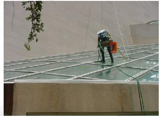
Water Infiltration Testing
