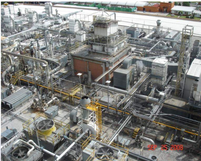
Food Mfg. Company; Queretaro, Mexico Roof Replacement Design/Administration
