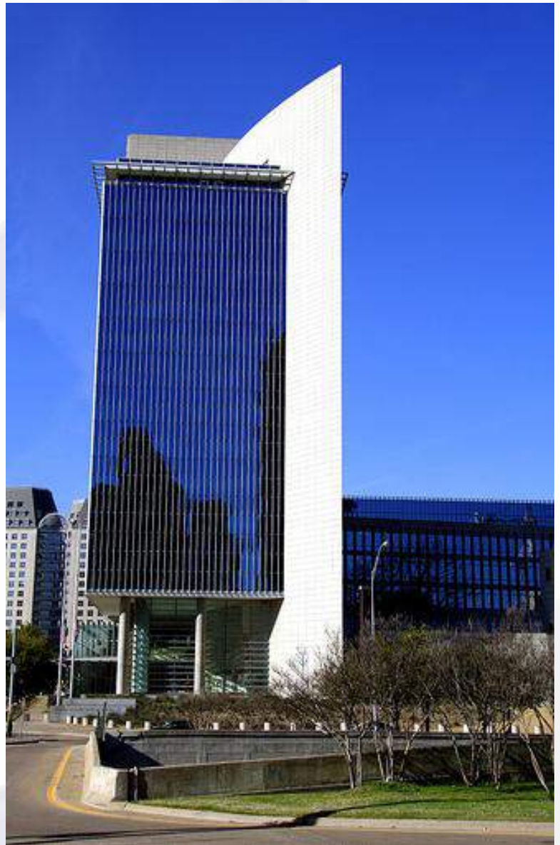
Federal Reserve, Dallas, Texas Roof, Wall, Plaza Restoration
