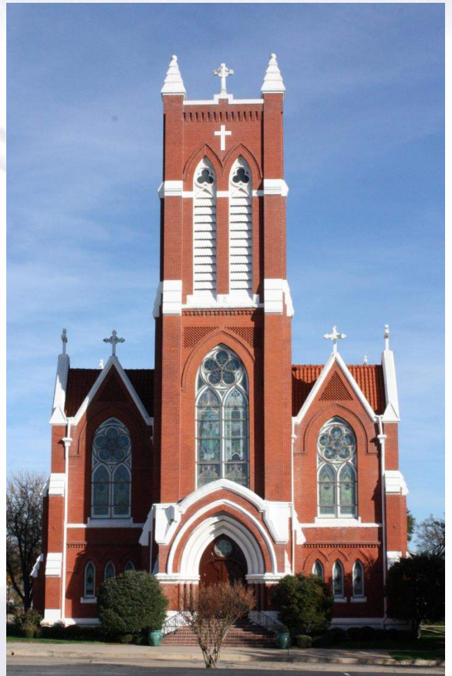
St Patrick Catholic Church Building Envelope Evaluation
